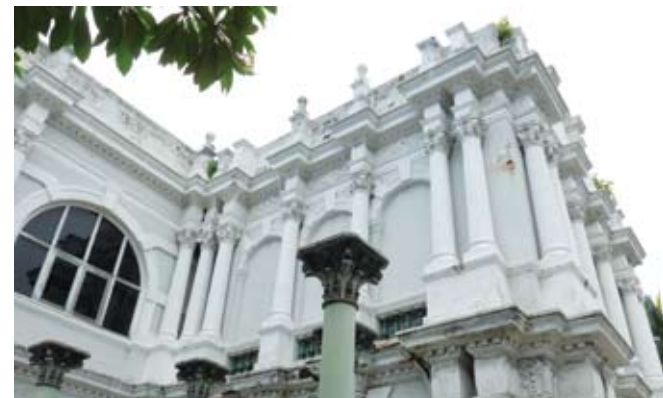
Penang Free School building in Farquhar Street.
